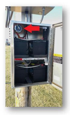
Turn off the battery disconnect switch.
